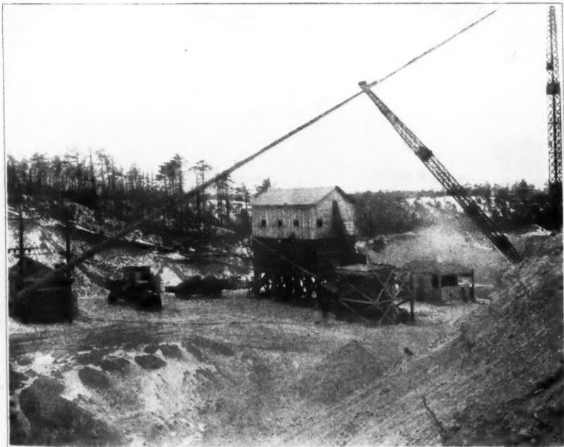
Notice the Approach to the Plant
